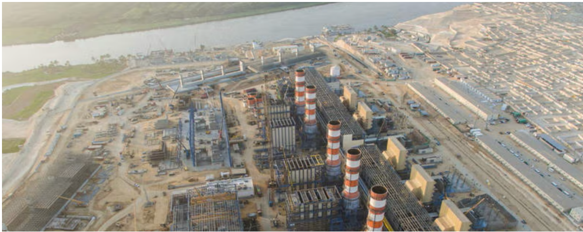
Siemens megaproject in Egypt (Adobe Stock)
